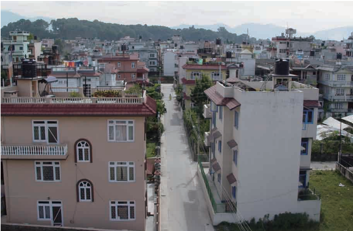
Figure 3.31. Residential development in Gongabu land pooling project area (2008) ▼
