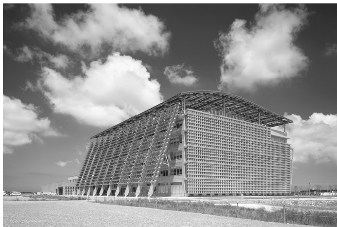
City hall equipped with a solar energy generation system on the roof and the wall facing south - Itoman City, Okinawa Prefecture
