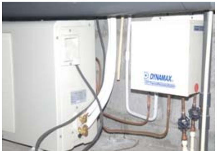
To minimize the energy consumption the resort uses air conditioners with heat recovery units, which convert the heat loss into hot water, in supplement to solar water heaters. In addition, a high efficiency dish washer with hot water connection is installed. Although with a smaller impact, energy saving lamps combined with solar lights are used. Energy efficient refrigerators and washing machines will be installed soon.
