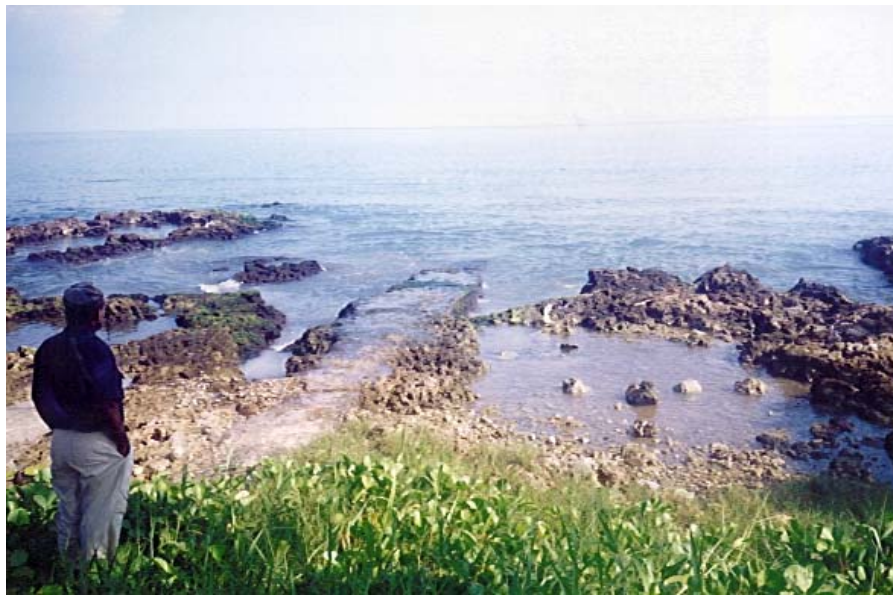
Photo 8.4: Typical ocean outfall in Honiara, Solomon Islands
