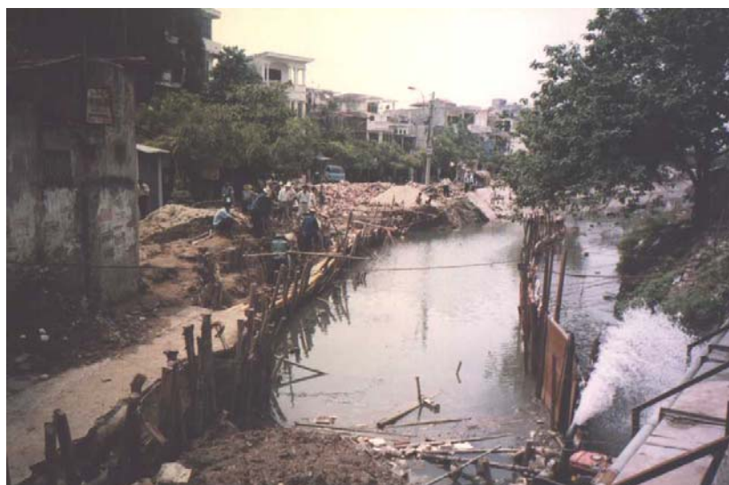
Photo 3.3: Kimnguu River under construction
