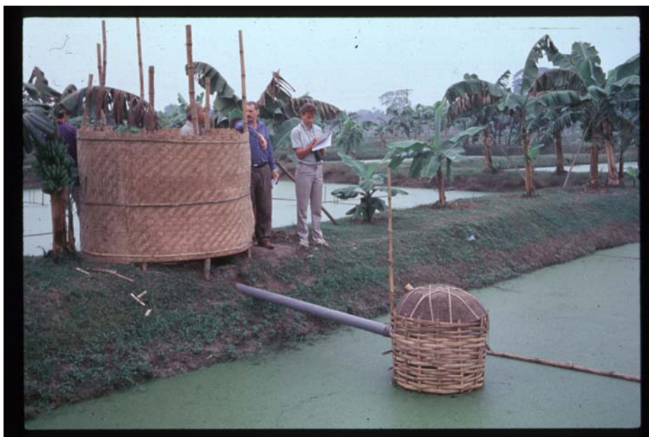
Photo 13: Demonstration of a nightsoil – fed duckweed system for rural households at Mirzapur, Bangladesh
