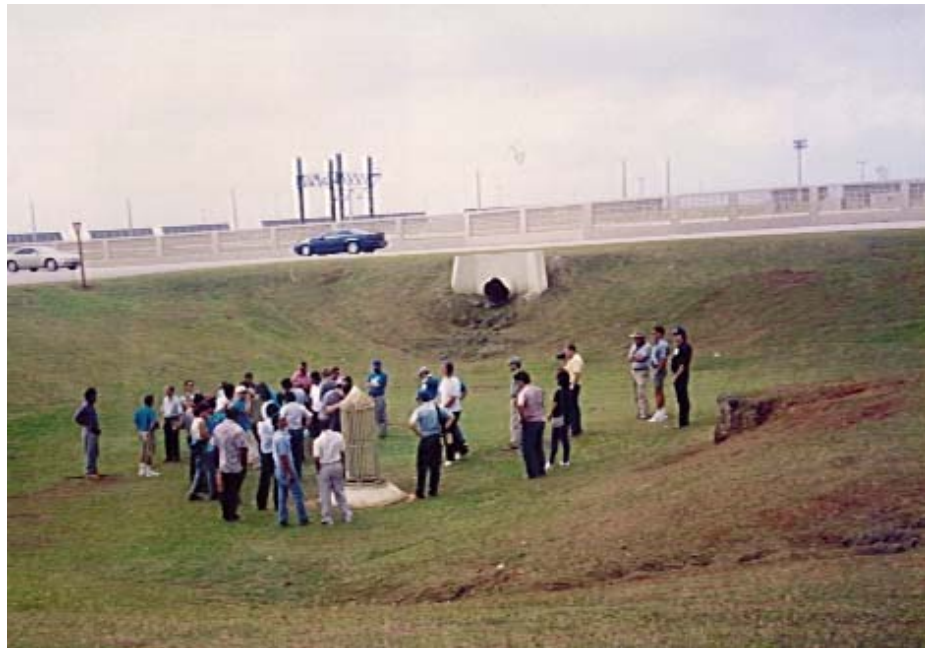
Photo 8.1: Stormwater disposal well in Guam
