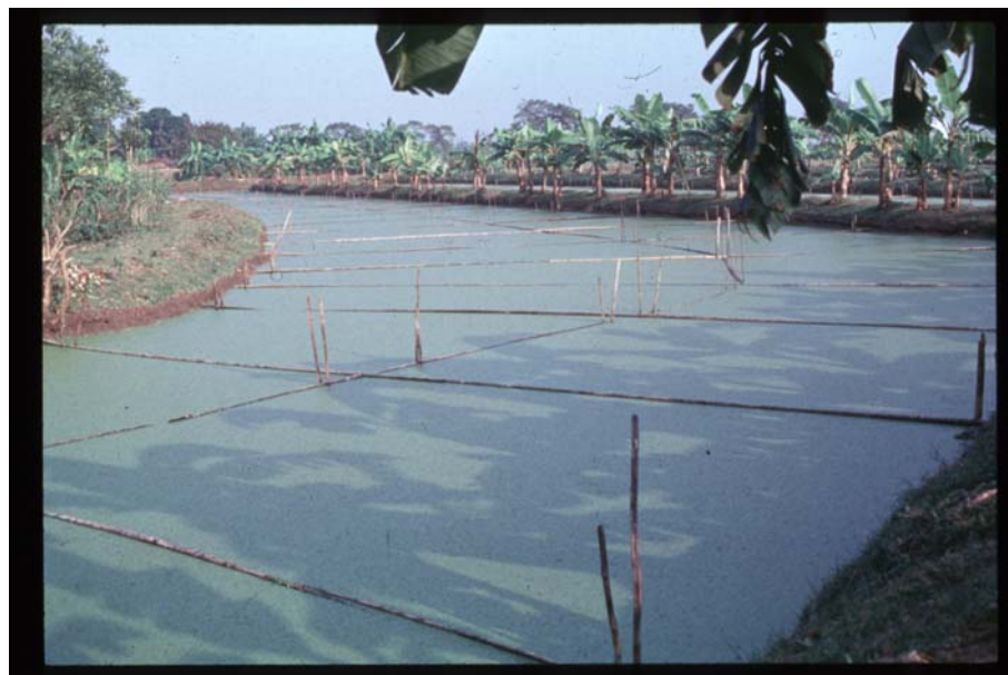
Photo 12: A duckweed based wastewater treatment system at Mirzapur, Bangladesh
