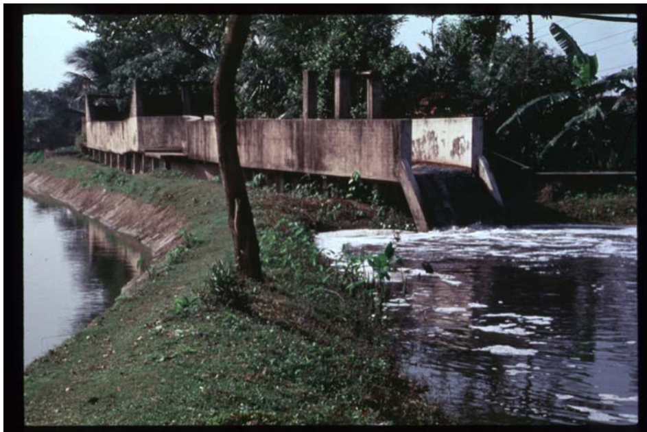
Photo 10: Pumping wastewater into an anaerobic stabilisation pond at Bandipur, West Bengal, India
