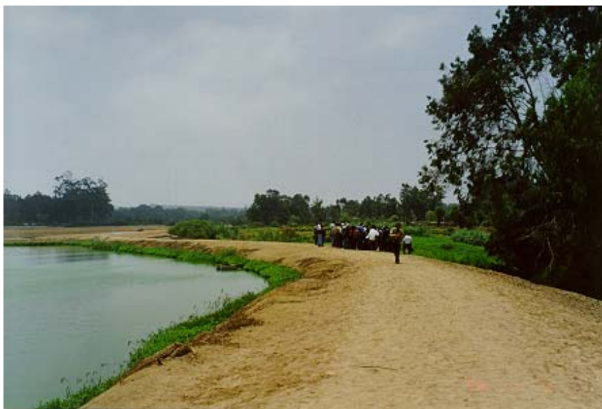
Photo 5.1: View from the treatment system (stabilization pond)
