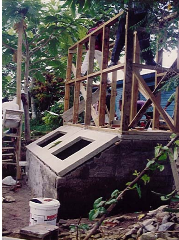
Photo 8.6: Construction of compost toilet in Fiji
